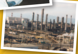
Los Angeles refinery work
